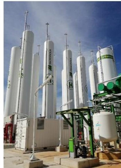
11 H2 storage tanks Supplied by IDESA and VAKO 60 Bars pressure ~4 tons usable capacity
