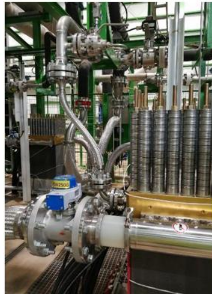
NEL ASA electrolyzer PEM technology 16 stacks of 1.25 MW each
