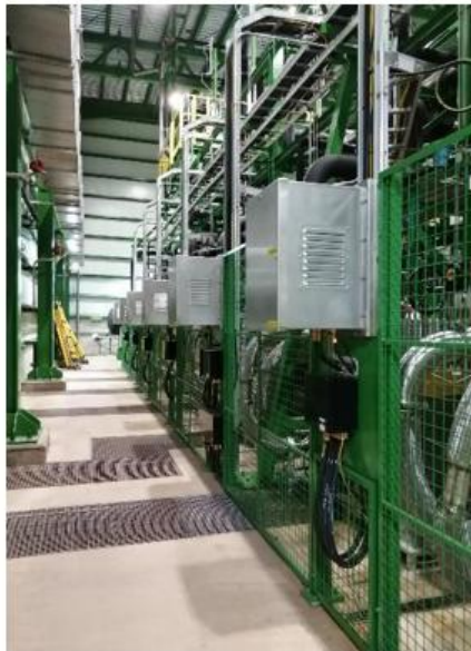
NEL ASA electrolyzer PEM technology 16 stacks of 1.25 MW each
